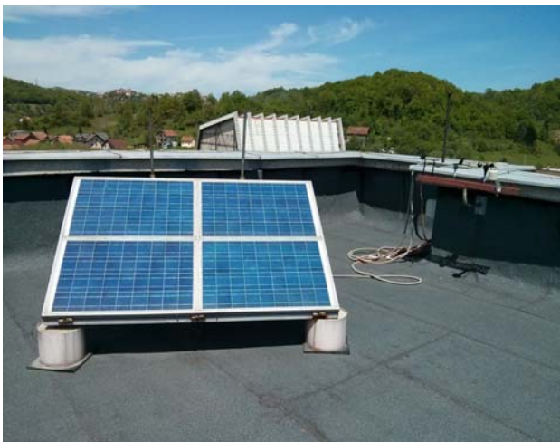
Figure 1. PV panels and weather measurement equipment mounted on the roof of Faculty
