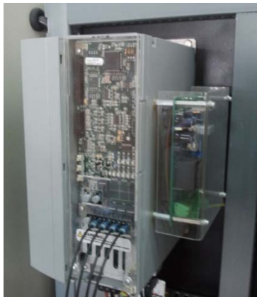
Figure 4. Standard industrial converter with integrated IPC card
